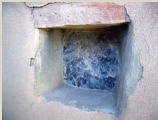
This is one of the last surviving mica windows which can be found at Acoma.
